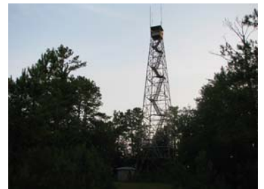
Remote radio repeater tower station and antennae.
